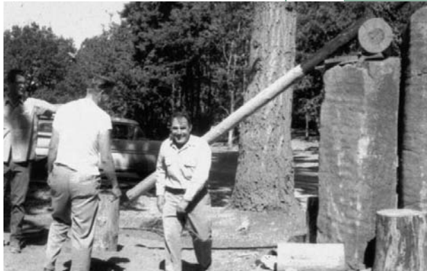
Placing pillars in 1967
